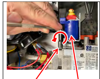
MANIFOLD PRESSURE TAP
