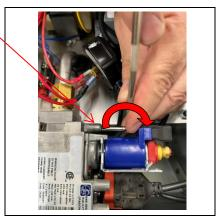
14) Replace the modulator plug and insert the screw.
