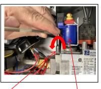
SERVICE DOOR GAS VALVE MANIFOLD PRESSURE TAP MODULATOR
