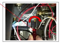
15) Replace the black plastic cap on the adjustment tower.
